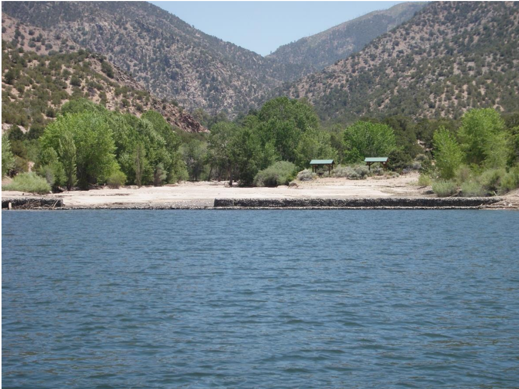
Figure 3 - Nambe Falls Reservoir retaining wall located in upper reservoir, June 2013.
